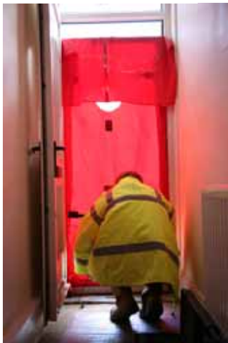
Setting up the Pressure testing door
