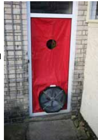
A Pressure testing door in situ
